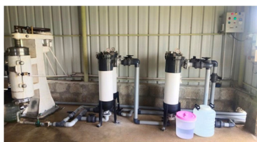
Tubular bowl centrifuge unit
